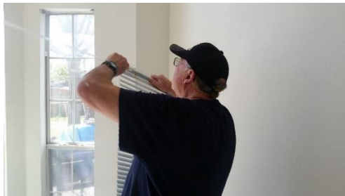
Rumsey repairing bay window at Chalko's
